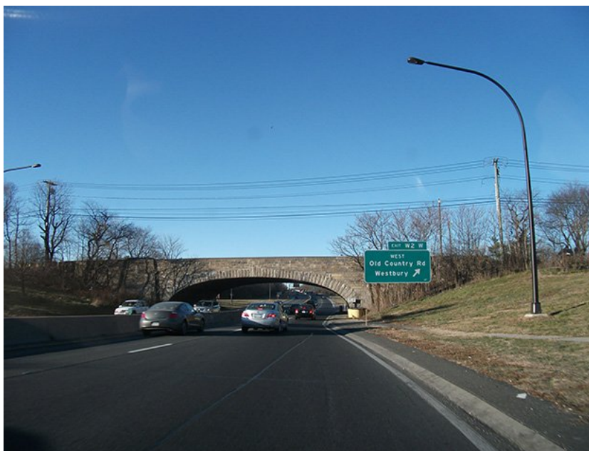
Low overpasses that public transit cannot pass through on Long Island Source: Doug Kerr via Flickr
