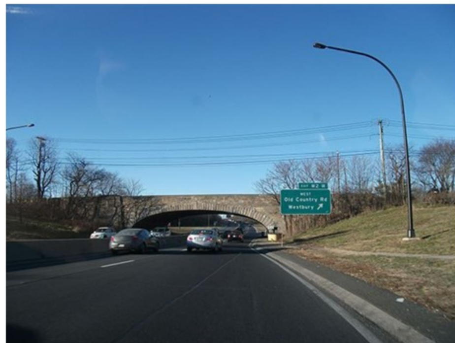
Low overpasses that public transit cannot pass through on Long Island Source: Doug Kerr via Flickr
